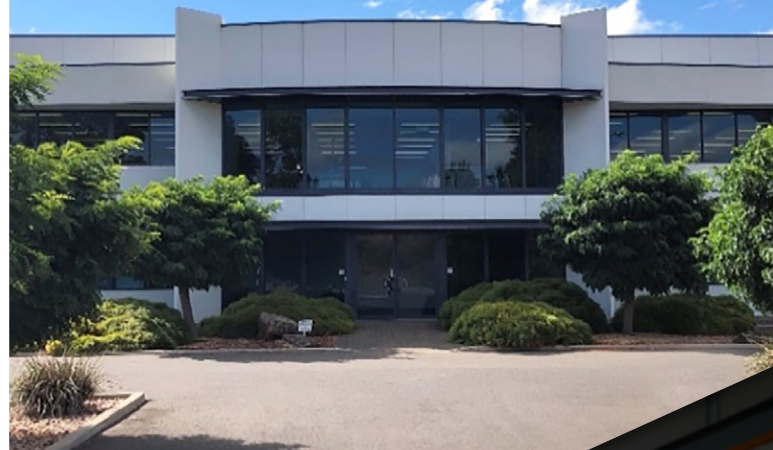
The new AML3D head office and manufacturing space in Edinburgh Parks, Adelaide.
