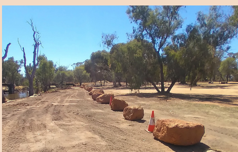
Image: River bank protection at Pumphreys Bridge
