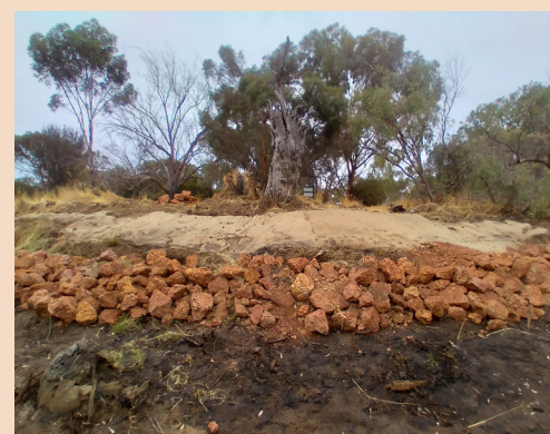
Image: Williams bank stabilisation (Planting on river bank to occur in winter)
