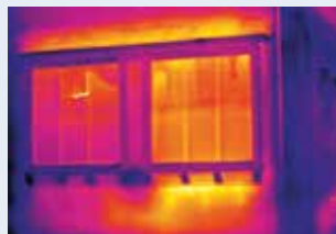
What a thermal imaging camera sees.
